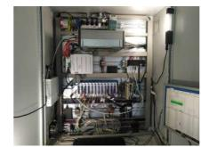
Central measuring station at tower base for recording and transmitting of all monitoring data
