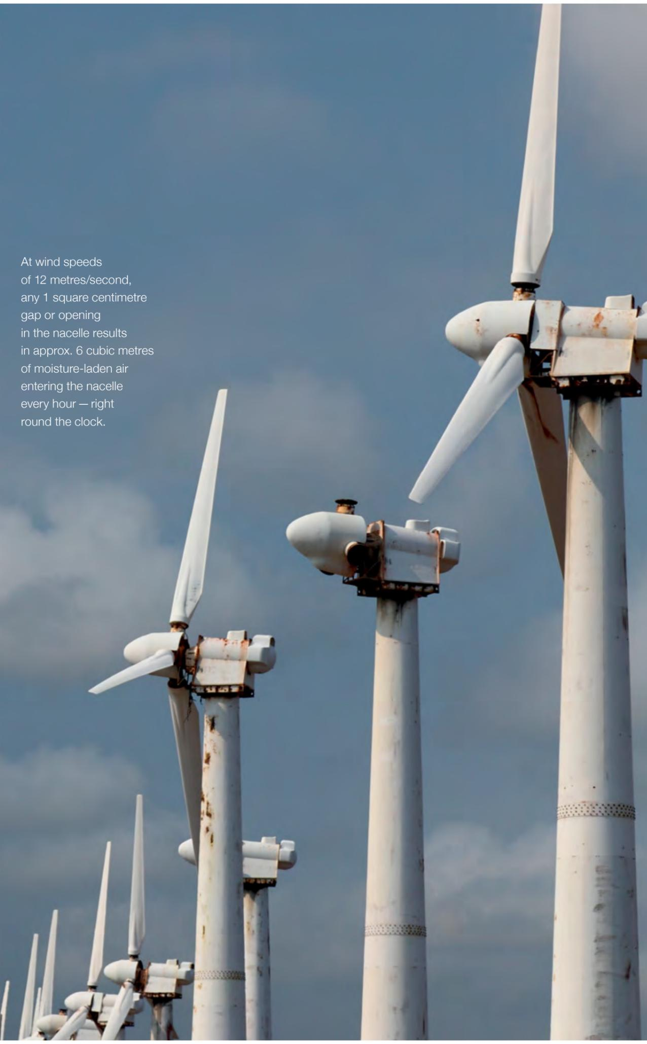
At wind speeds of 12 metres/second, any 1 square centimetre gap or opening in the nacelle results in approx. 6 cubic metres of moisture-laden air entering the nacelle every hour — right round the clock.
